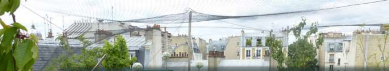
On the roof of a research institute in Paris; Foto: Runrid Fox-Kämper
